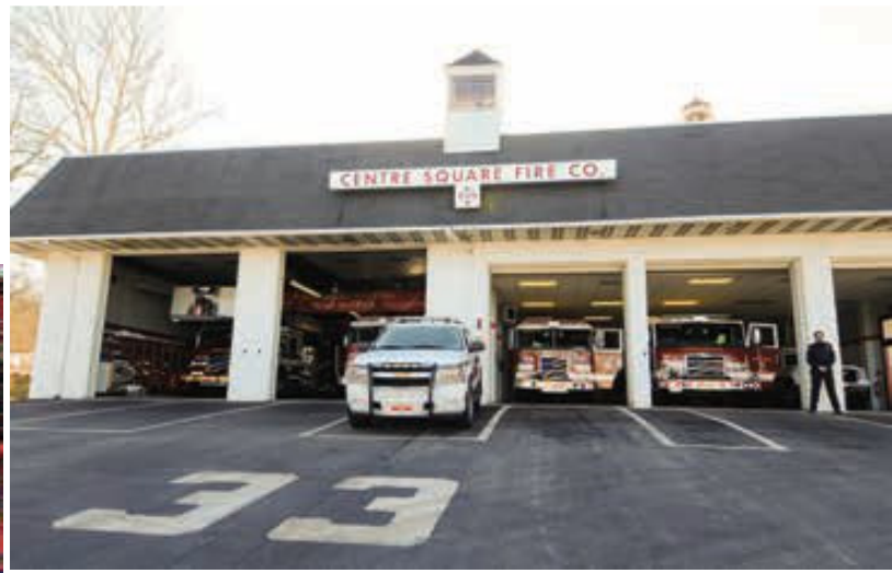
CSFC33 Fire Station, Circa 1954. Construction on a brand new fire house will begin in June 2016.
