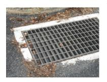
2.Replace storm sewers in the parking lot of the building. This project includes new storm piping and storm inlets. With the paving of the parking areas over the past years, water had been too often routed to the foundation of the building; water now is directed to the storm sewer. This project will protect the building's foundation. Work was done by the Whitpain Public Works staff.
