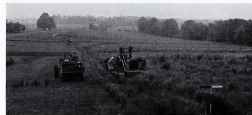
Digging the trench for the ceramic tile drainage pipe shown in the truck on the left.
