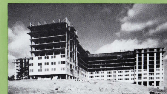
Chetwynd Apartments at midway point during construction. The aluminum skin was erected at 2200 square feet daily rate.
