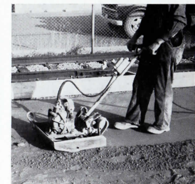
Bed prepared for concrete slab, Nov. 13.
