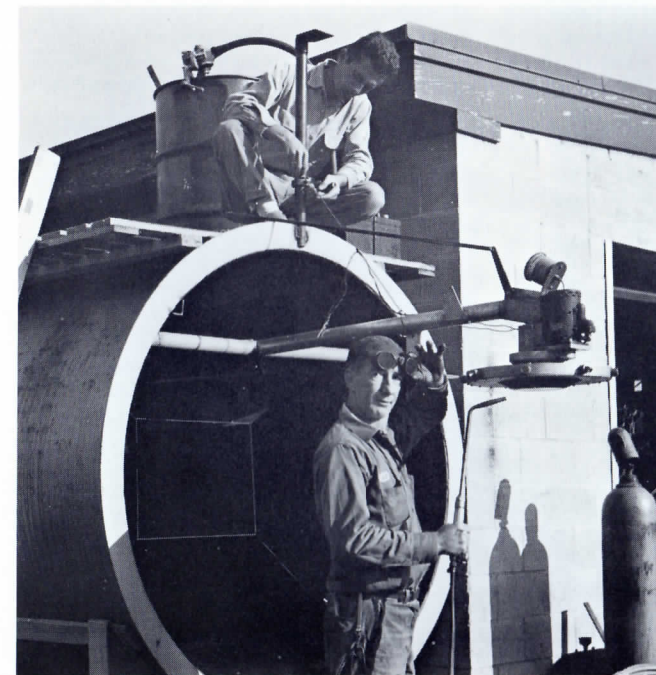
Special iron wind tunnel was designed and erected to duplicate actual spraying conditions while testing efficiency of different types of nozzles. Harold McKenzie (standing) has just completed welding sprayer to tunnel; Joe Mallozzi is adjusting valve on the feed tube. Propeller is off U.S. Navy "Drone" used as target.
