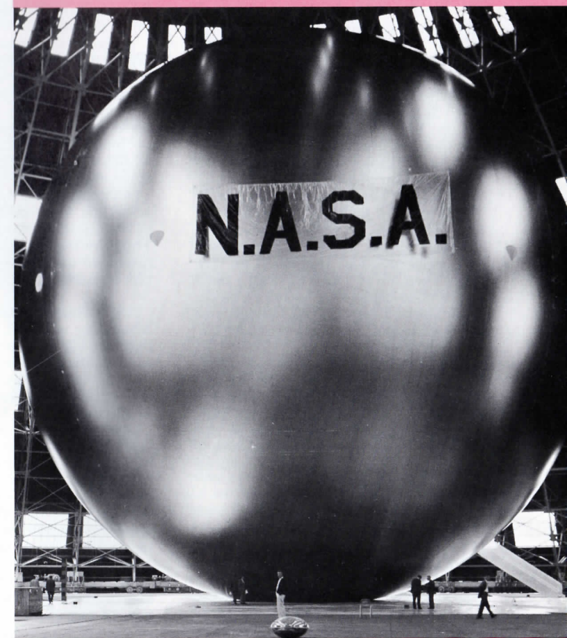
This 135-foot inflatable balloon satellite is expected to be put into orbit by National Aeronautics and Space Administration in communications experiment. Amchem was requested by NASA to produce Alodine chemical coating for similar satellites. This chemical is now being tested.
