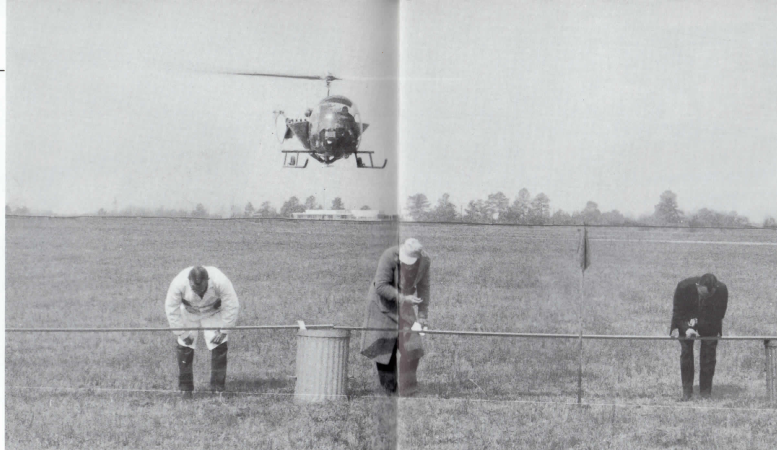
Counting Aqua Kleen granular after it was applied by TVA helicopter with Amchem-designed sprayer rig in calibration run at Muscle Shoals.
