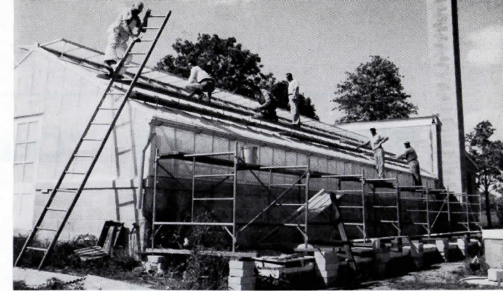
Buildings and equipment are always kept in tiptop shape. Here the greenhouse is being completely weatherproofed by installing Alodized Aluminum bar caps at the glass joints. Work is performed by maintenance crew under supervision of FRANK PIACITELLI: (l. to r.) Norm Chestnut, Johnny Zollo, Bob Wright, Piacitelli, Harvey Burrell and Andrew Lawrence.
