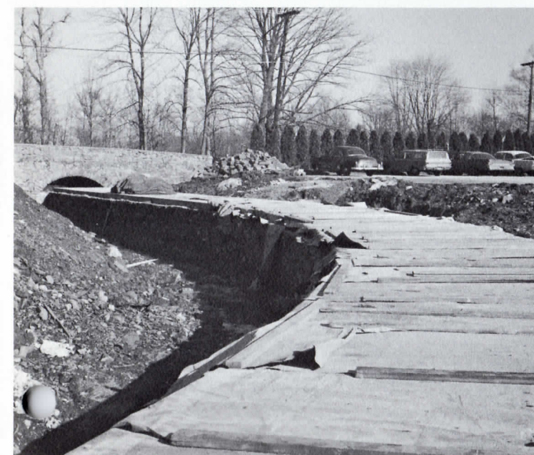
Curving roof of viaduct is made of reinforced poured concrete.
