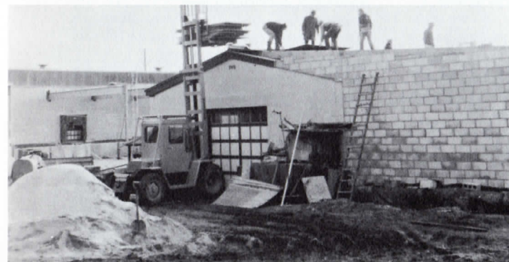
Group installing plywood on roof. Note use of new fork lift truck.
