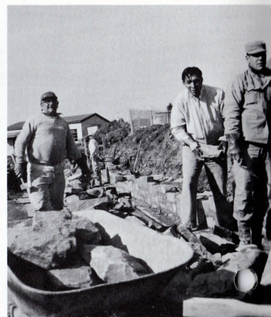
Constructing cut stone side walls of viaduct.
