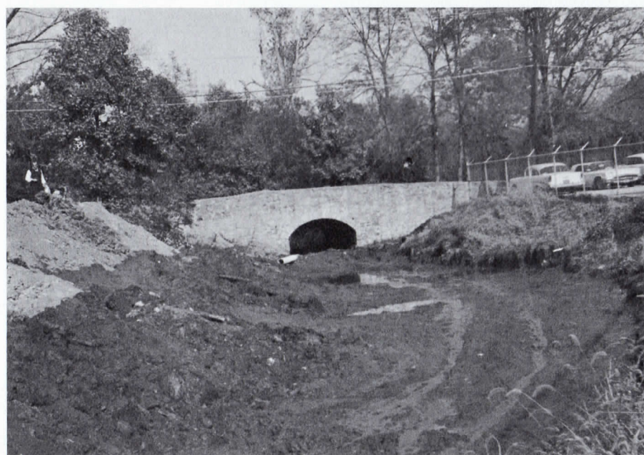
Diverting flow of creek by creating temporary new bed before building side walls.
