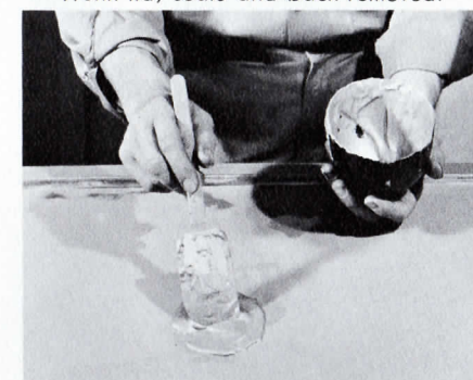
Plastic-metal fills damaged spots.
