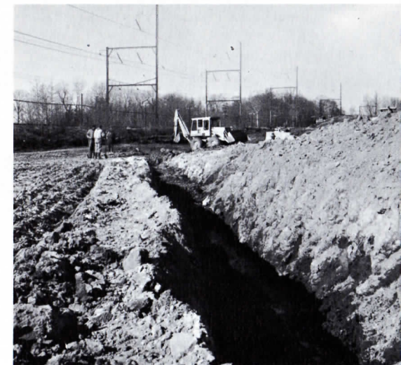
Waste water line had to be relocated.
