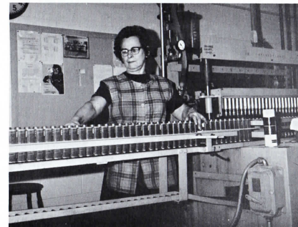
Fannie Cram feeds pint-size cans to automatic can filling machine. Machine fills 48 cans of this size per minute.
