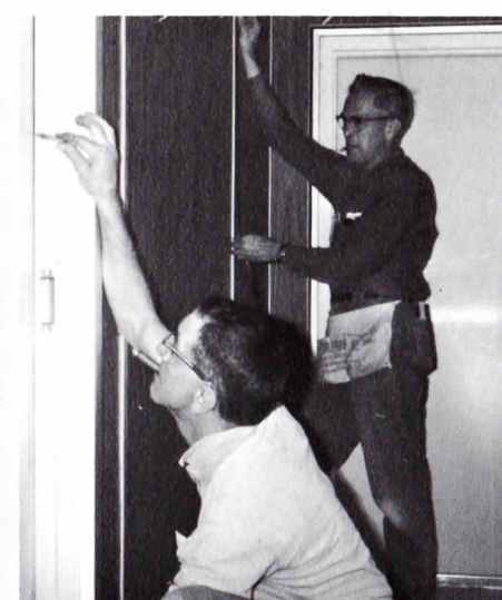
Tony and Ed Wood assure doors and molding strips fit perfectly between panels.
