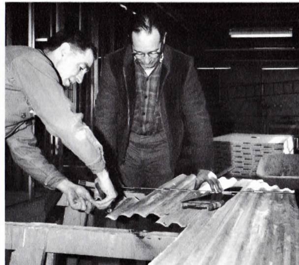
Tony and John trim galvanized corrugated base covering steel joists before concrete is poured for floor.
