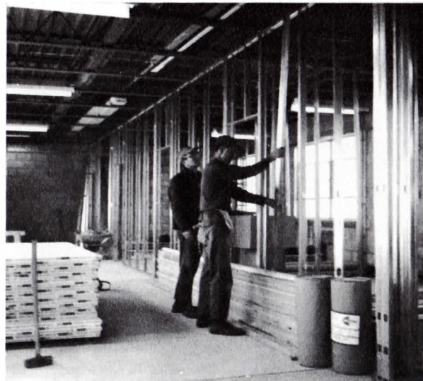
Skill and ingenuity displayed in creating new ACD offices. John Piacitelli and Tony Serratore plumb studding.
