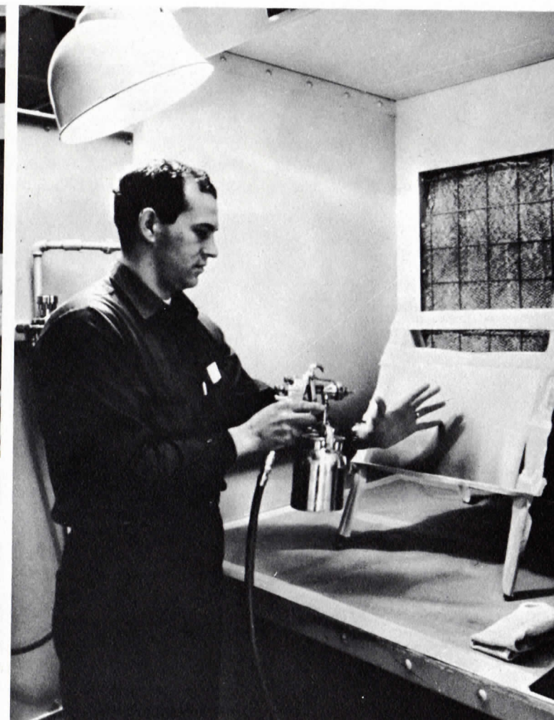
Student at shop class tests distance between panel and spray gun.
