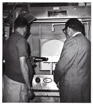
Doug Blosser demonstrates newest technique for applying organic (paint) coatings in powder form by electrostatic spray.
