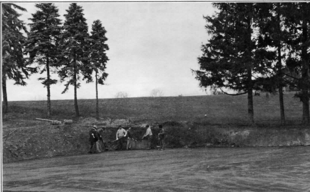
This little group from Frank Piacitelli's construction crew is part of Frank's work force that cleared away 2,200 cu. yards of rock and earth, and paved a new section for outdoor storage of materials.
