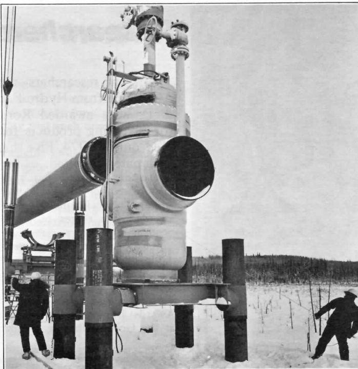
One of the trans-Alaska pipeline projects that was completed during 1974 was this pipeline block valve demonstration section north of Fairbanks.
