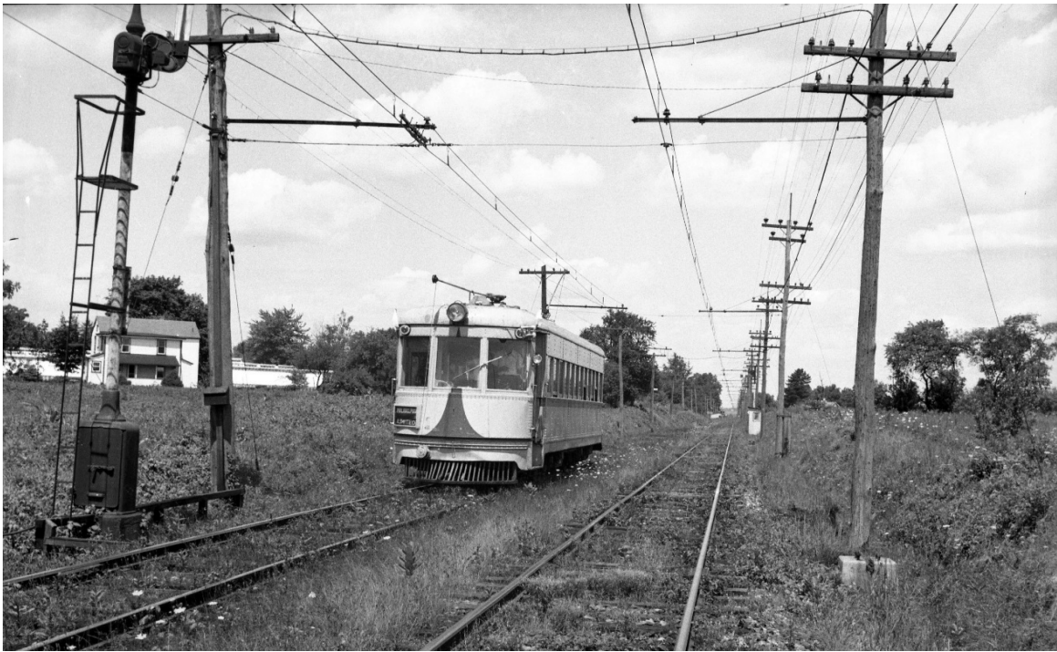
This southbound trolley waits at Acorn Siding, between Township Line Road and Morris Road. Passing sidings such as this were essential on what was for most of its length a single-track railroad.
