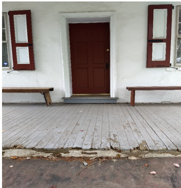
Deteriorating flooring at the Franklinville School's front porch, October 2021
