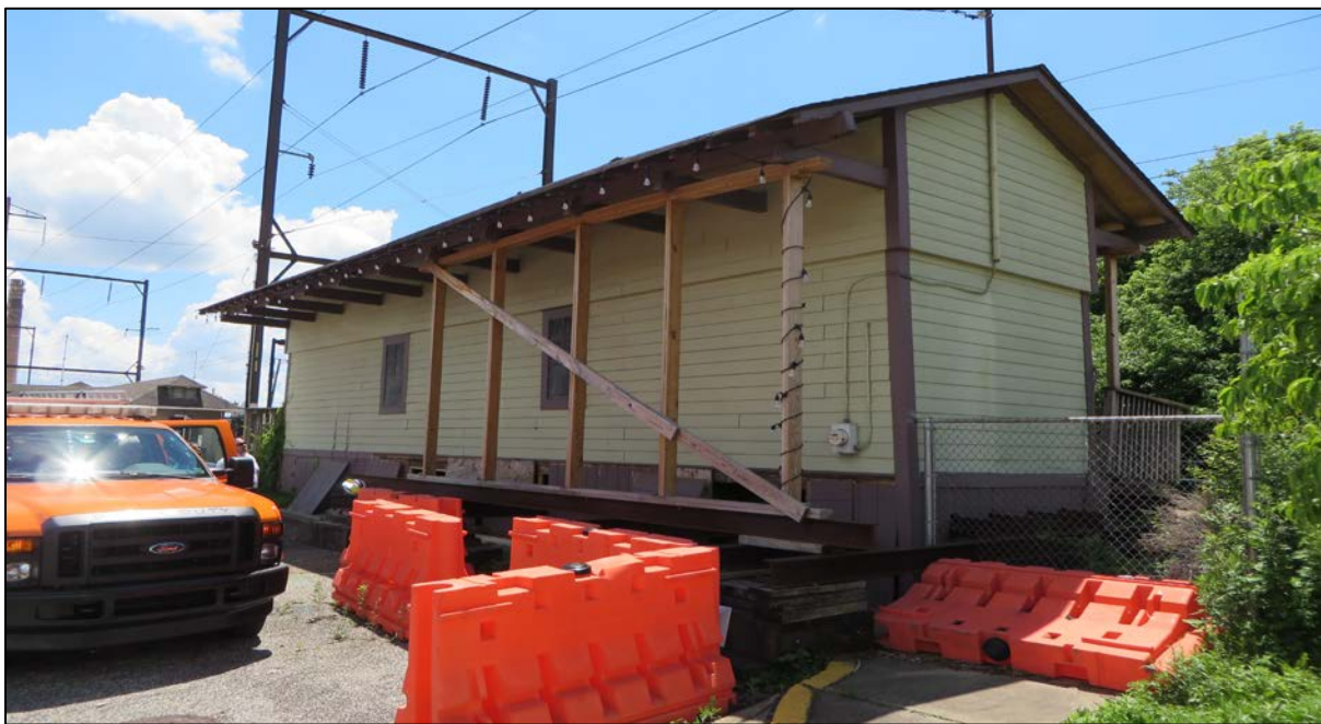
Photo from SEPTA, showing the reverse side of the Freight House. The orange barricades obstruct a cavity under the building. (May 2022)
