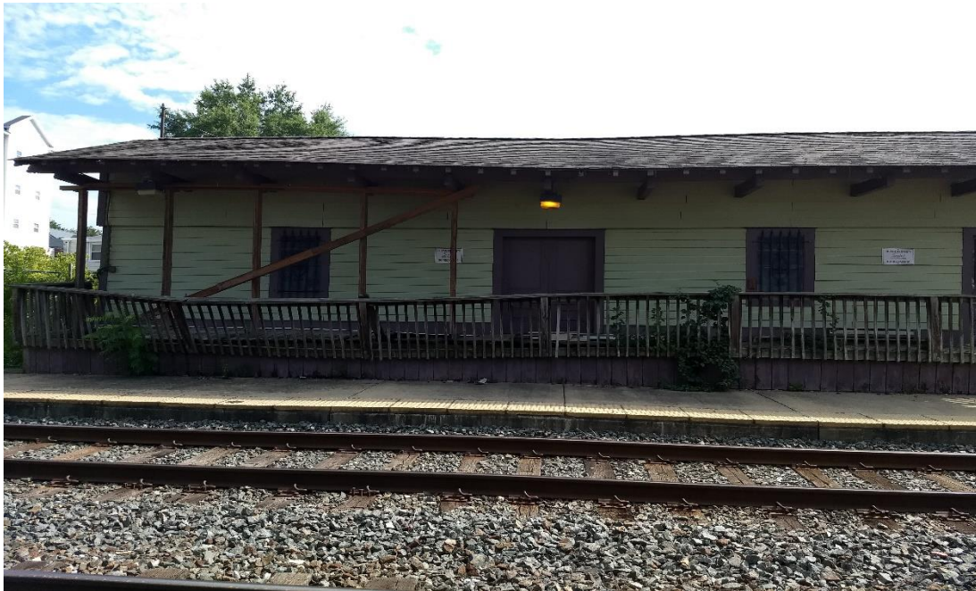
The 1875 Freight House with sagging floors due to water damage.
