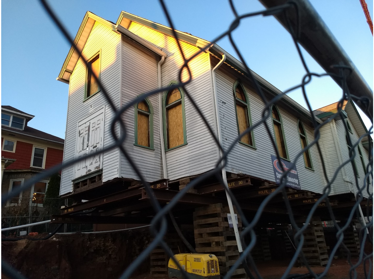
The Colony Club's building, once a church, was raised on temporary "stilts" for renovation. Soon to become a condominium, according to the county, it is an example of "adaptive reuse."
