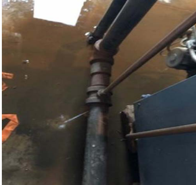
At the 1895 School's furnace room, water spurts from a leaking pipe onto the wall. (The white rectangle above is a light fixture.)
