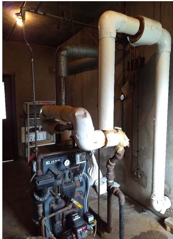
The repaired heating system with new, covered pipes.
