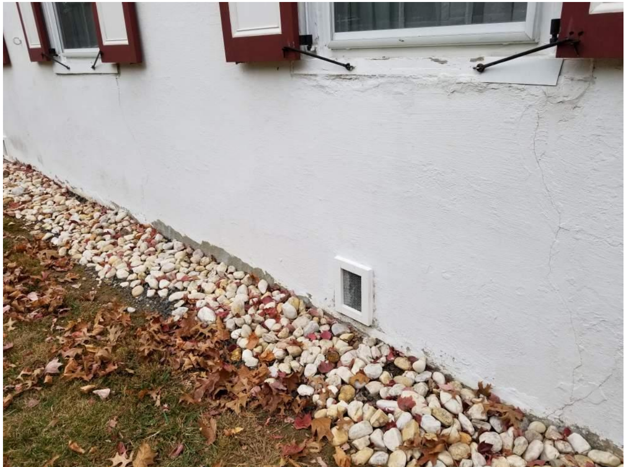
At the Franklinville School, one of four screen-covered vents to the crawl space under the floor, recently restored by Steve Vereb. Note the cracked stucco under the window.
