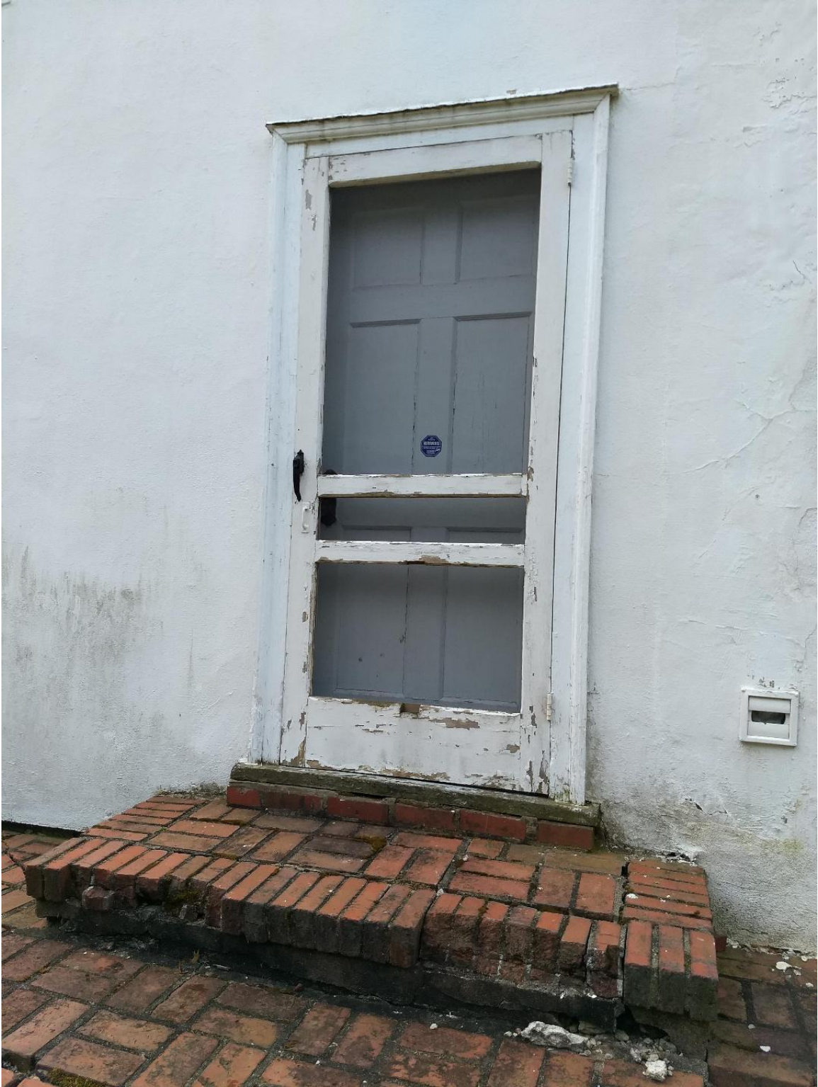
The back of the 1858 Franklinville School, the 1930s addition, with peeling paint and leaking stucco (Photo from April 2023)
