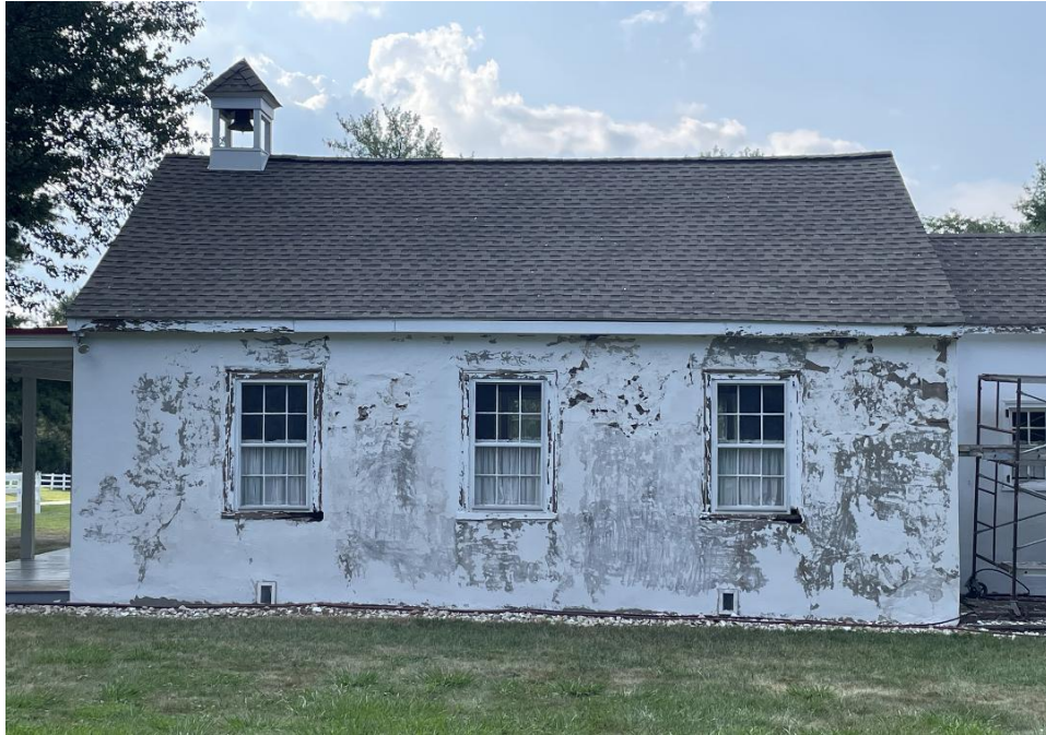
The side of the Franklinville School after loose stucco was removed, August 18, 2025 (Photo from Barry Johnson)
