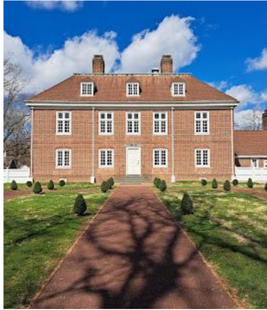
Pennsbury Manor, built 1683
