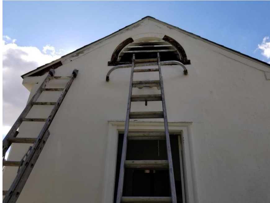
Work continues on the vent over the back door, Oct 27, 2025
