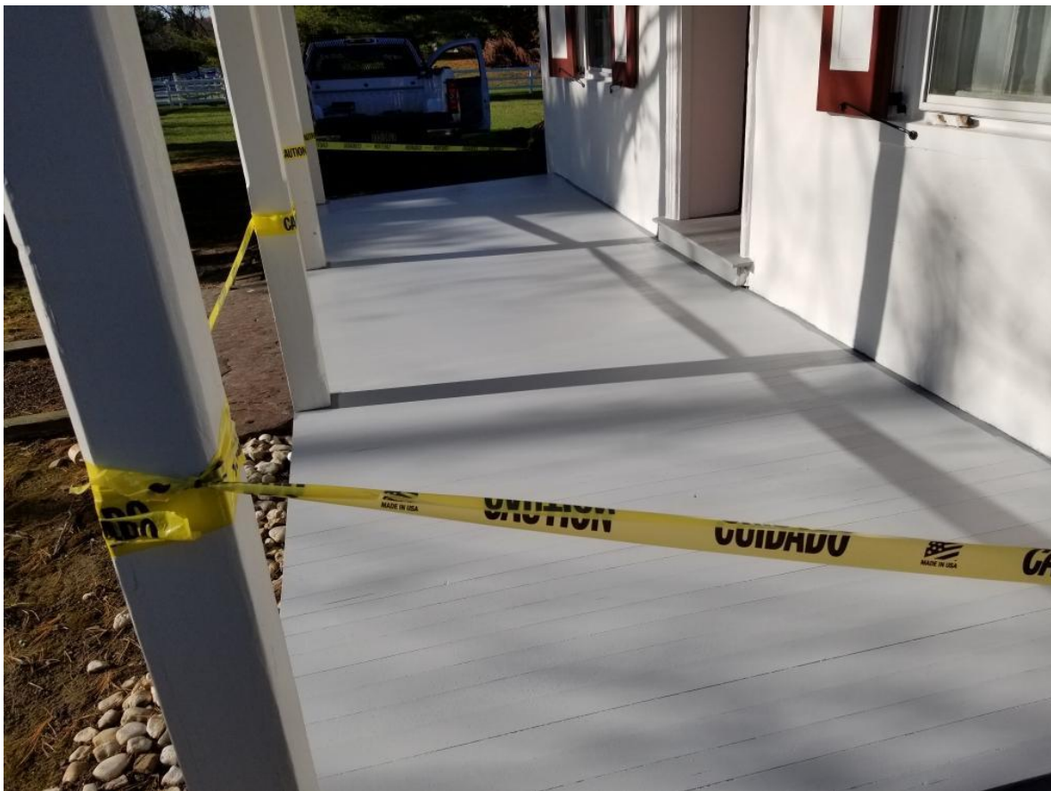
Newly painted front porch, Nov 11, 2025
