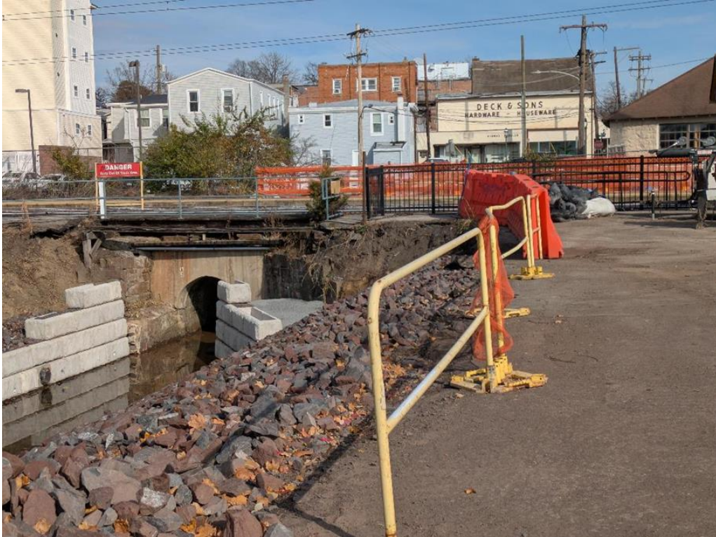
At Ambler Train Station, where the Freight House used to stand, work on the culvert will continue. A metal liner has been ordered (Photo, Nov 7, 2025).
