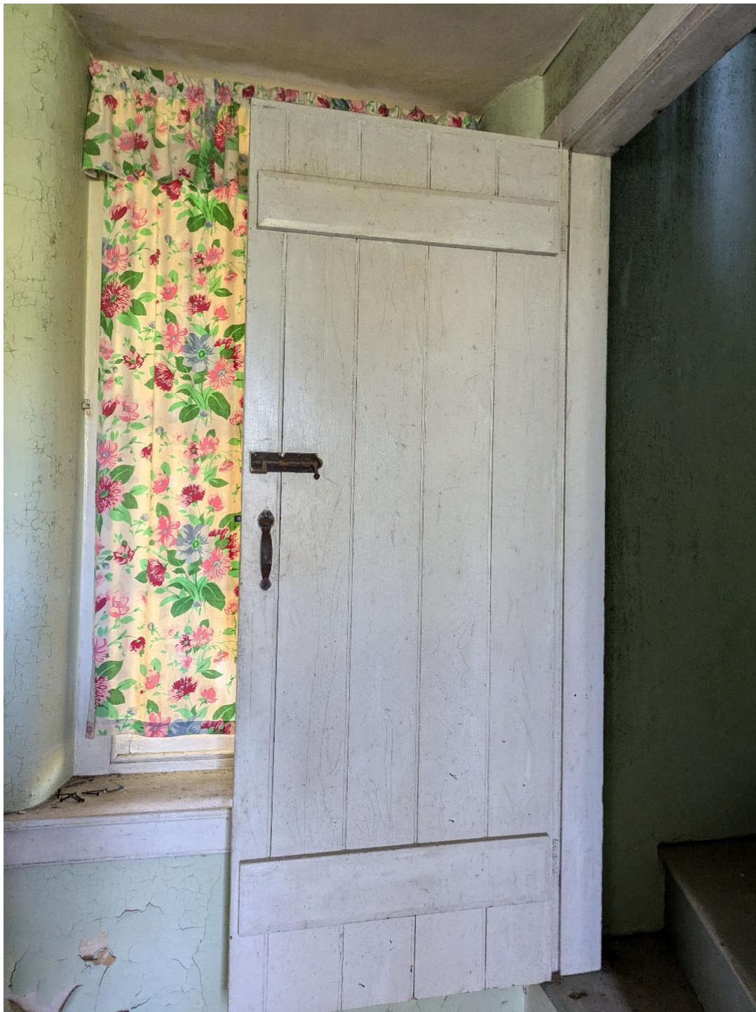
At the "Homiller House," the board-and-batten door, typical of houses built in 1830-1850, with its original hardware. Note the peeling paint in the lower left of the photograph.
