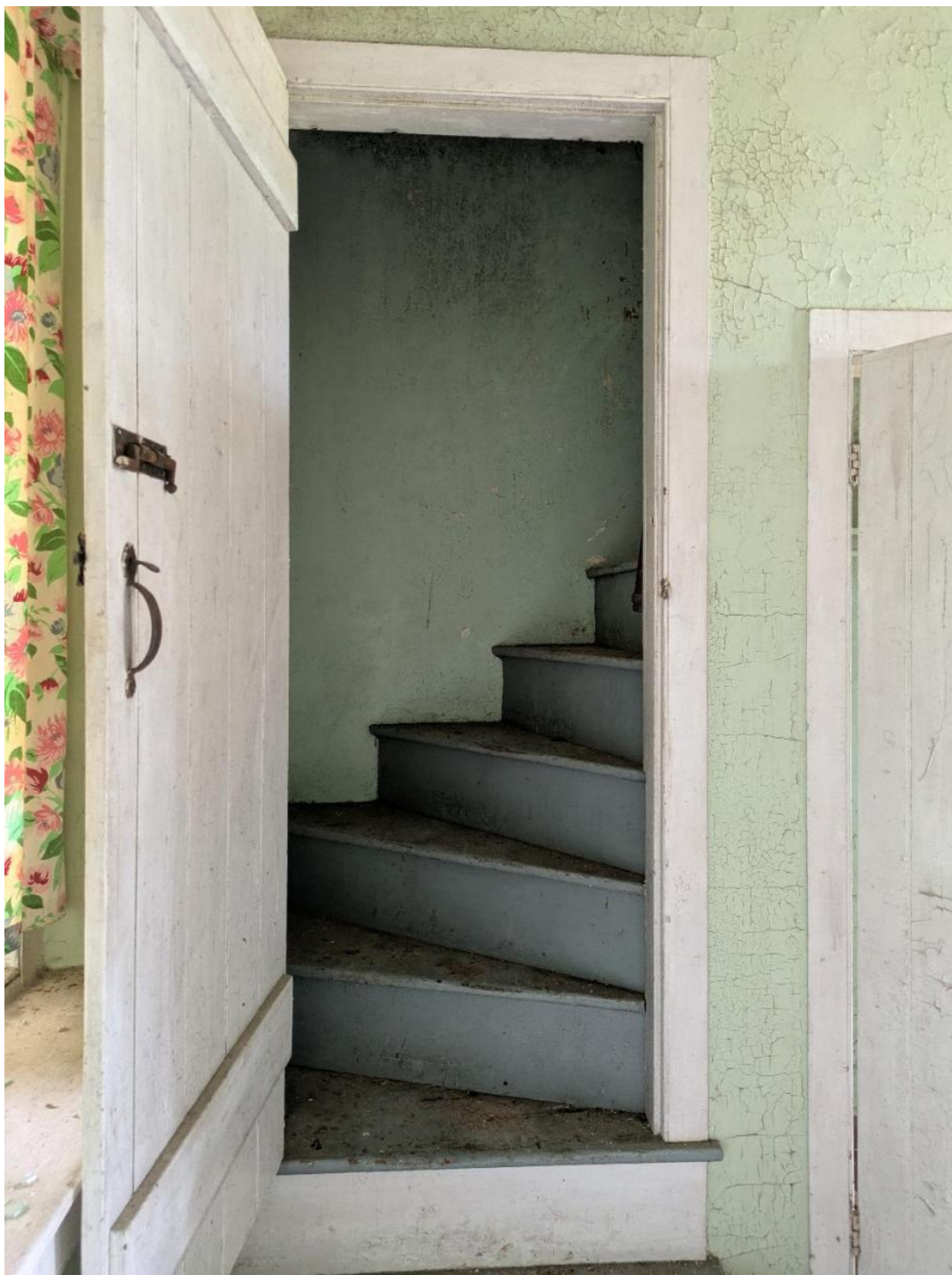
Back stairs from the kitchen to second floor. Note the floral curtain fabric on the left. Its remnants appeared in a later pile of rubble. Note also the old board-and-batten door. This photo was taken on the day before the tear-down.
