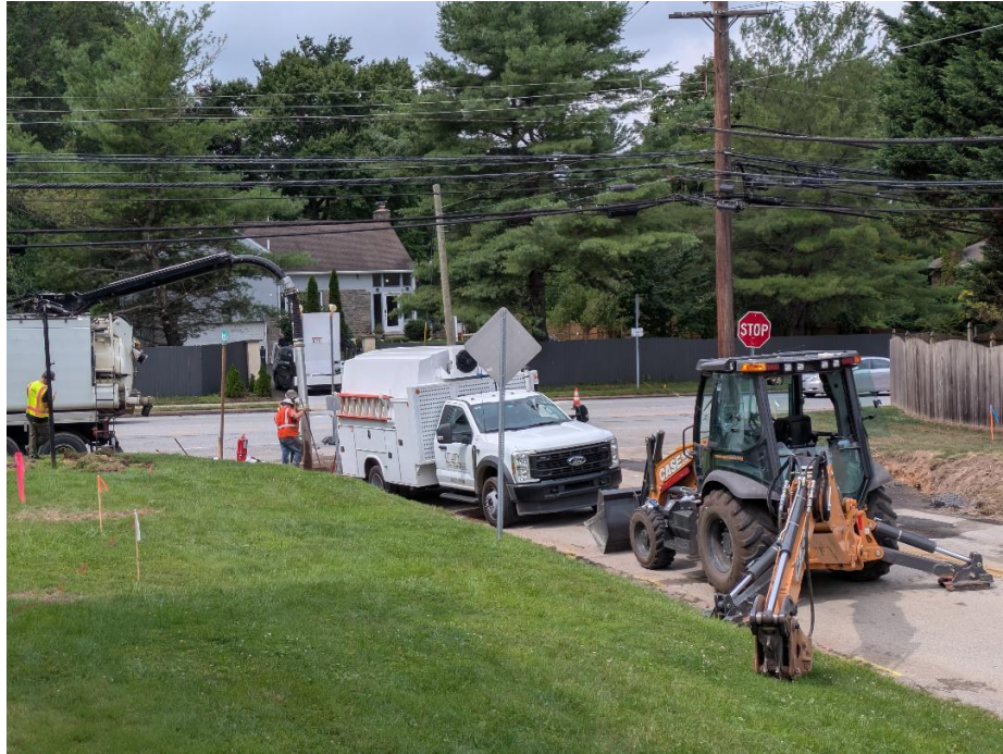
To begin the project, workers cleaned the drain at the corner.
