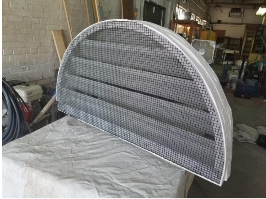
The back of the vent with screens to keep out insects and squirrels
