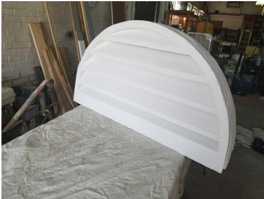
Photo by Steve Vereb, proud craftsman who rebuilt the attic vent cover at the Franklinville School. Precise work demanded. He had to bend the wood (spring 2026).
