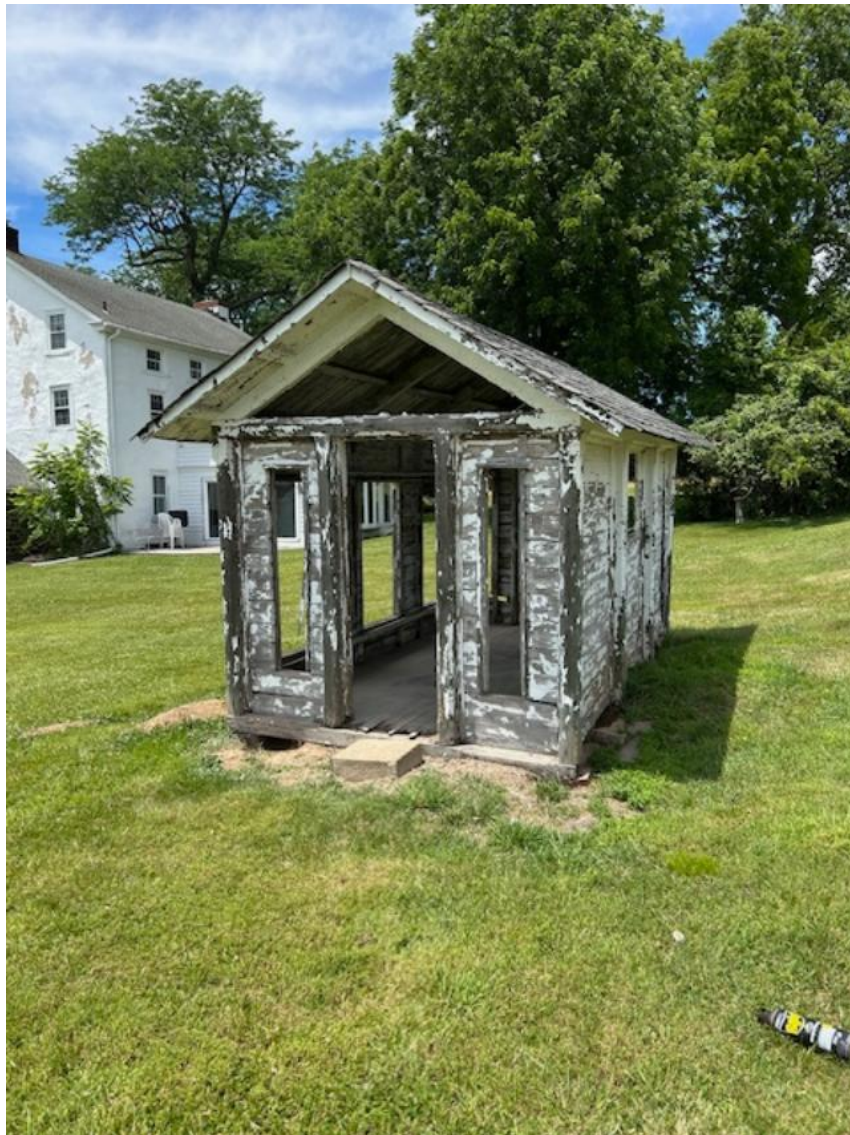
The Skippack Pike Toll Booth with windows and doors removed
