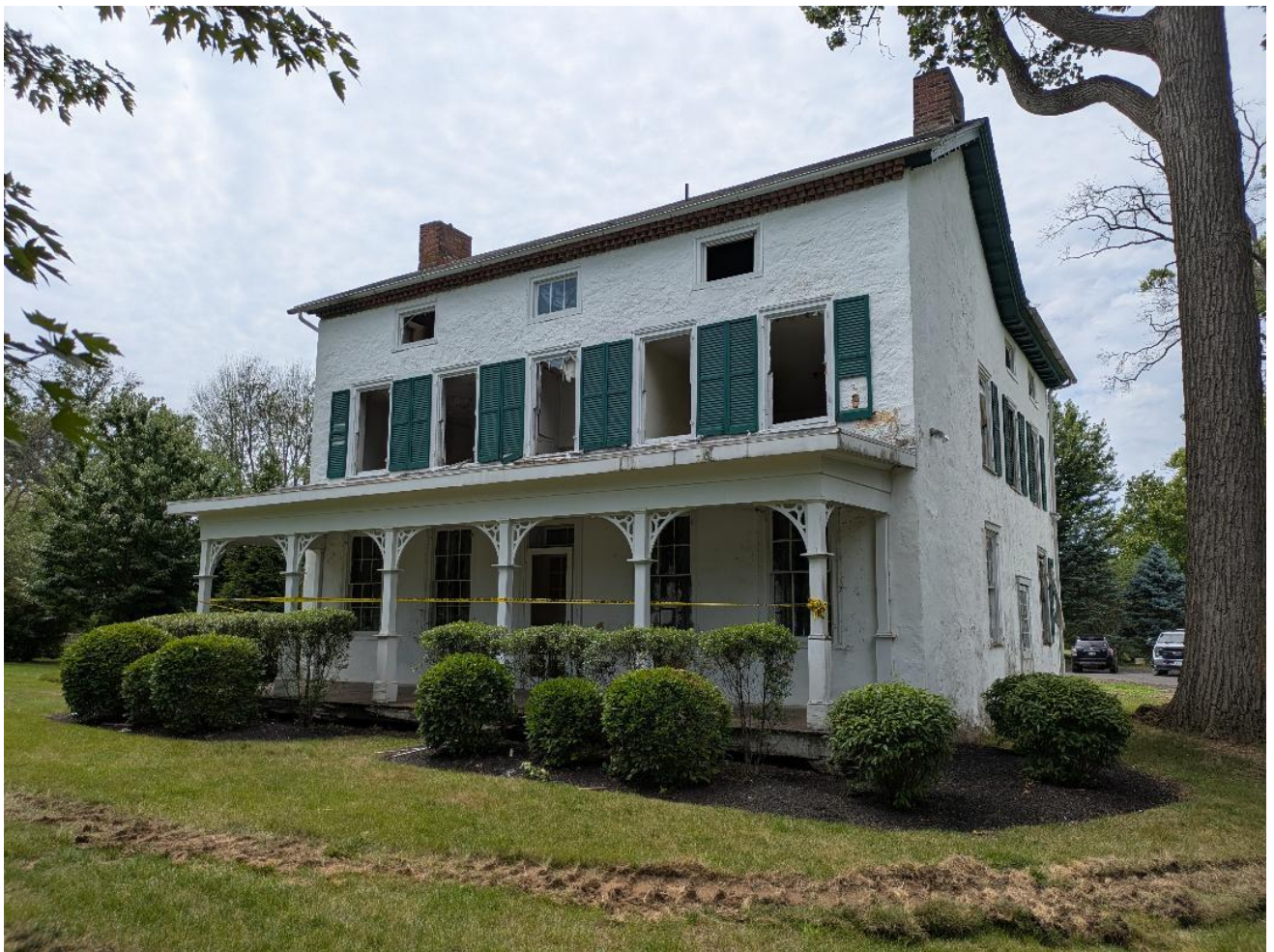
The Homiller House on Tennis Avenue with its windows removed. (Old glass is sold online for property owners replacing the glass at historic structures.)
