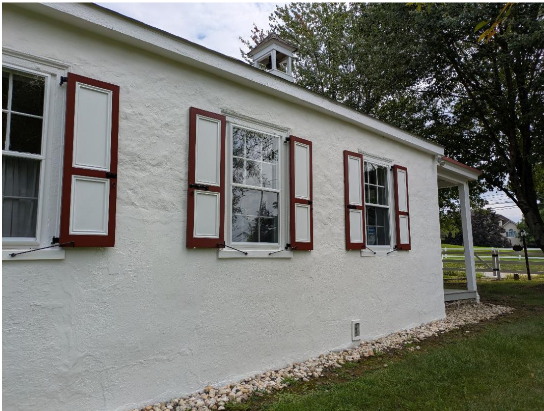
Newly-painted exterior wall and shutters at the Franklinville School, August 18, 2026
