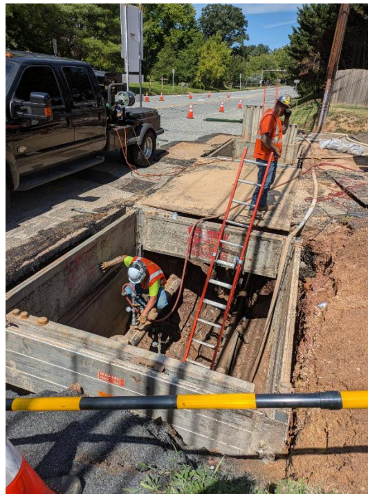
Underground work along Skippack Pike at School Road
