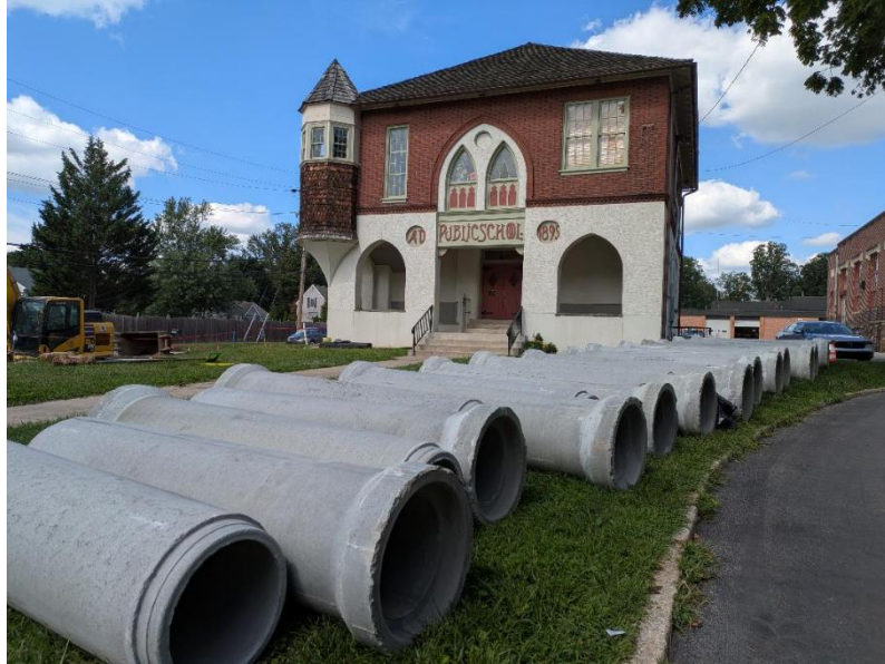
Got pipe? These are concrete drainage culverts that will be installed along School Road (August 16, 2026)
