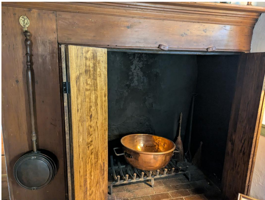
The walk-in fireplace at local home built in 1714
