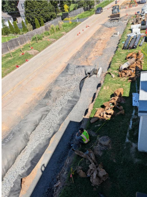
Workers added gravel on top of the membrane.
