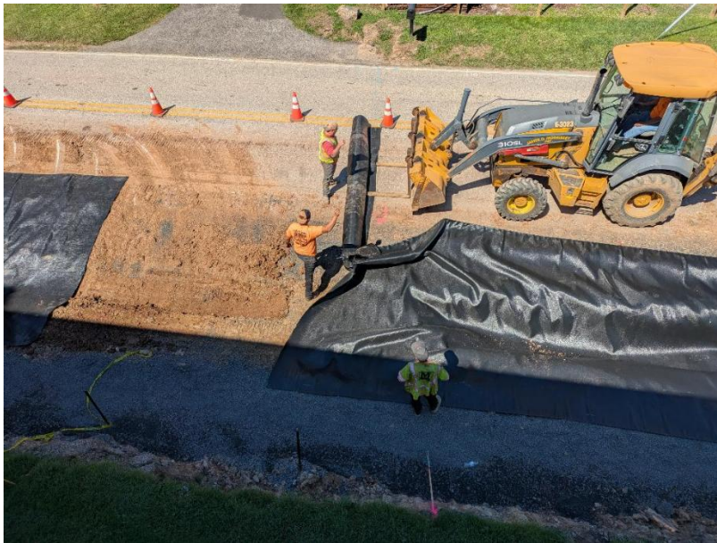
Workers unrolled heavy black material, a waterproofing membrane, to cover the soil along the new lane of School Road.
