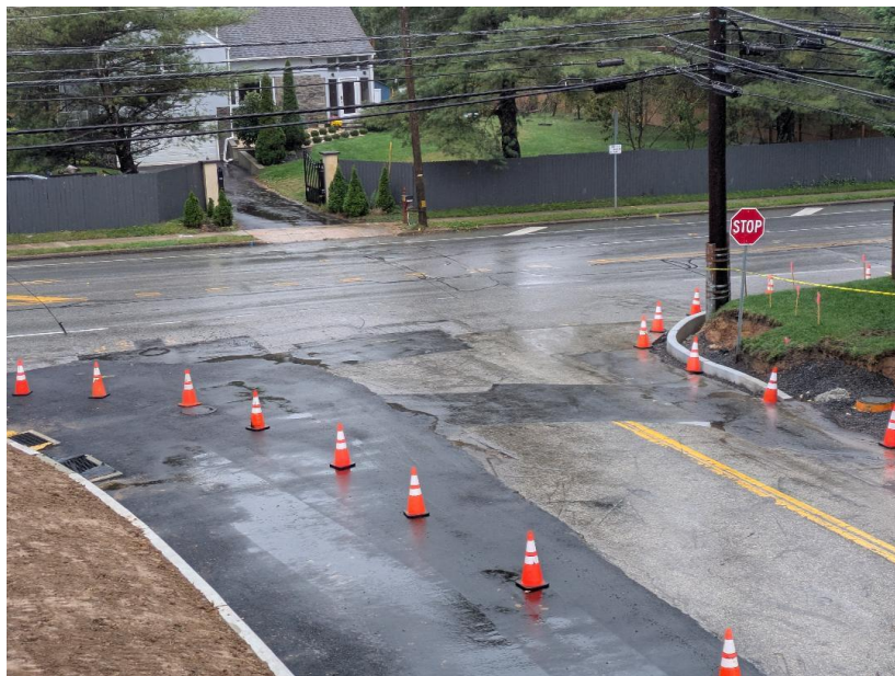
The intersection of School Road at Skippack Pike will be a lane wider than before construction.
