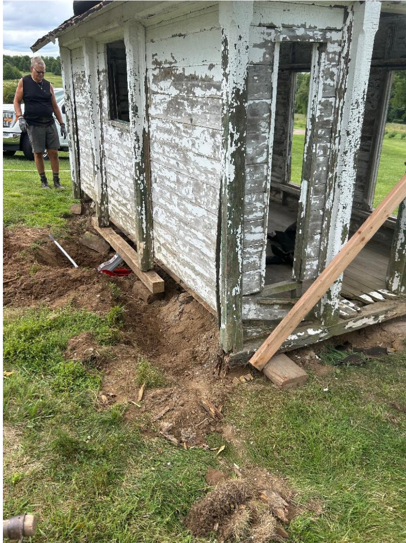
Member Larry Mulligan, preparing to lift the Skippack Pike Toll Booth, so it can be moved to solid ground for restoration
